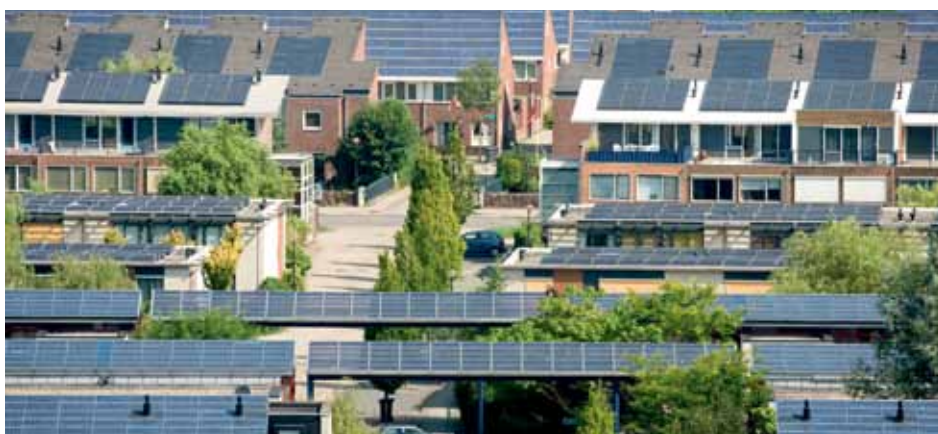
A PV project totalling 1 MW on the rooftops of the town of Nieuwland, Amersfoort district. Up until 2016, residential installations represented more than three quarters of total Dutch PV capacity.
